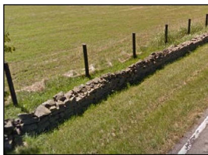
Site 10, Drylaid Stone Wall
