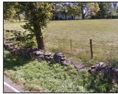
Site 7, Drylaid Stone Wall
