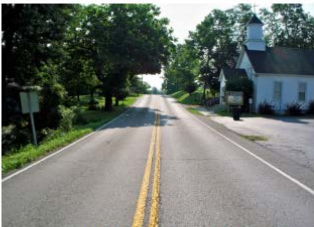
US 460 Looking East near MP 1.55
