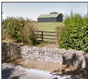
Site 15, Drylaid Stone Wall
