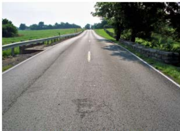
US 460 Looking East near MP 3.60
